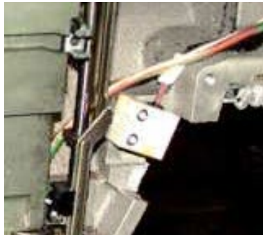
Figure 1 Laser Assembly Installed
