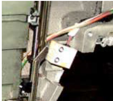
Figure 1 Laser Assembly Installed
