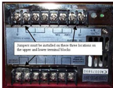
Figure 2 - Power Supply Unit Terminal Jumpers
