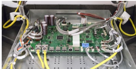
Figure 1 - Main PCB Installed
