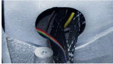
Figure 3 - Left Lower Arm Access Hole
