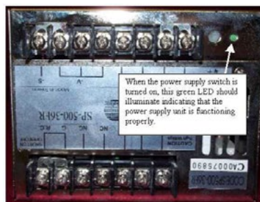
Figure 3 - Power Supply Indicator LED
