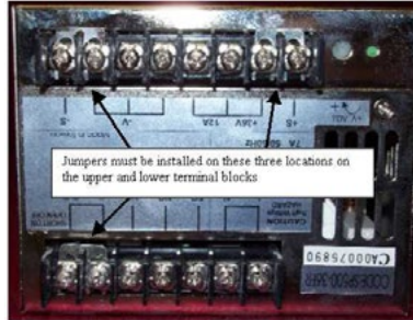
Figure 2 - Power Supply Unit Terminal Jumpers
